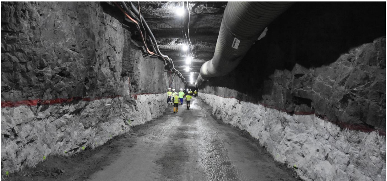
Figure 4: Kundu Decline; Electrified and Ventilated
