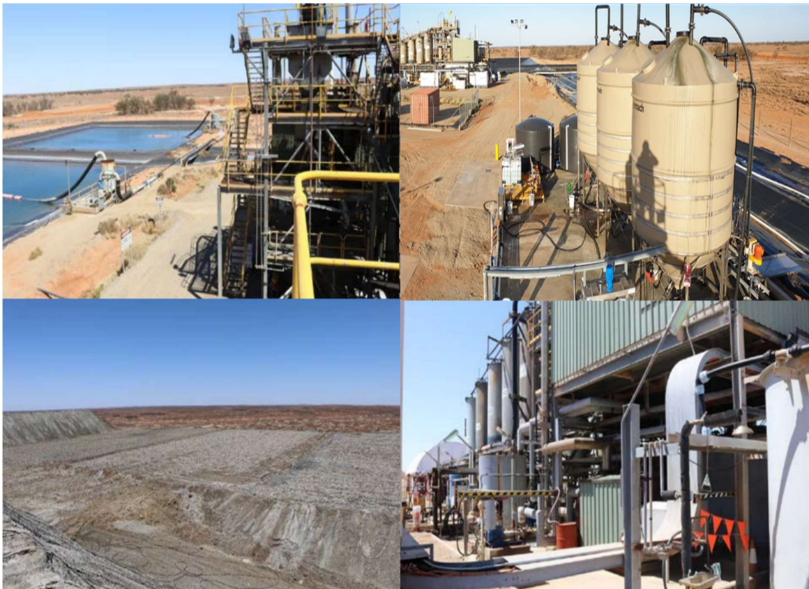
Figure 14: White Dam Gold Plant and Associated Infrastructure.
