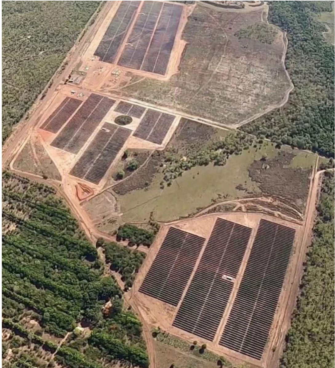
Figure 6 Solar farms at Batchelor (Batchelor 1 and Batchelor 2) adjacent to the Winchester project
