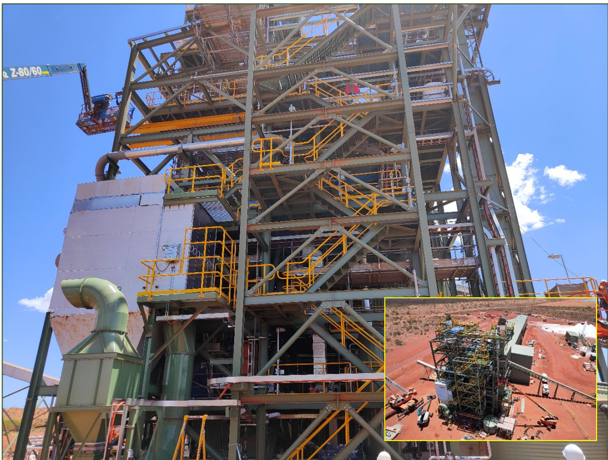
Compaction Plant Near Completion
