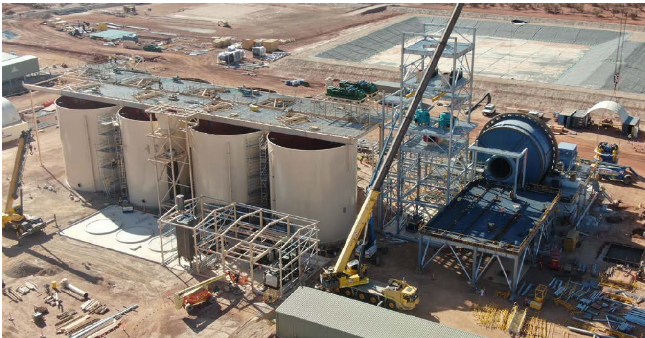
Figure 1: SAG mill shell, motors and girth gear now in position.
