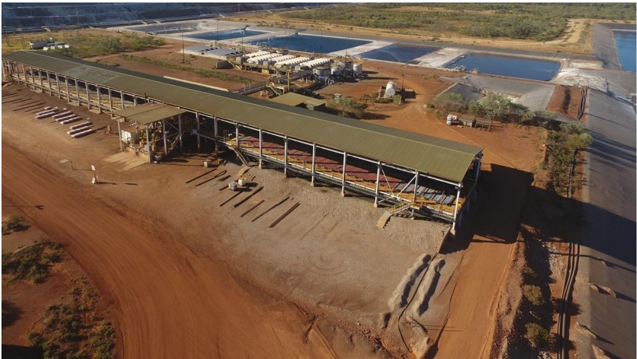
Figure 9. Mt Kelly electrowinning tank house in foreground and solvent extraction circuit in the background.
