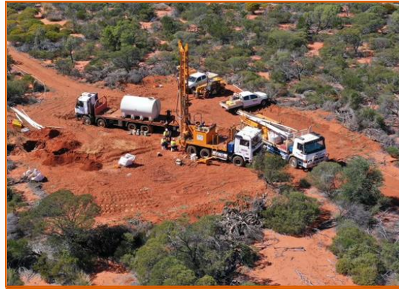
Water Monitoring Bore Installation
