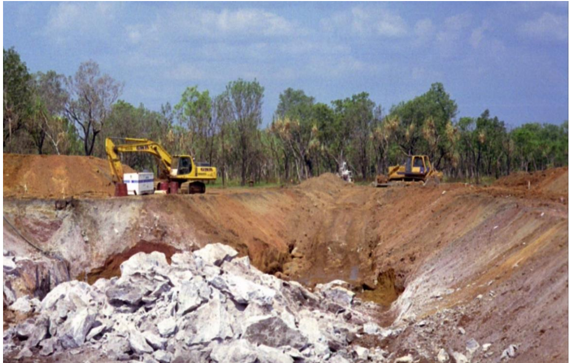
Figure 2 Test mining of magnesium at Winchester during the wet season (after blasting Level 0)
