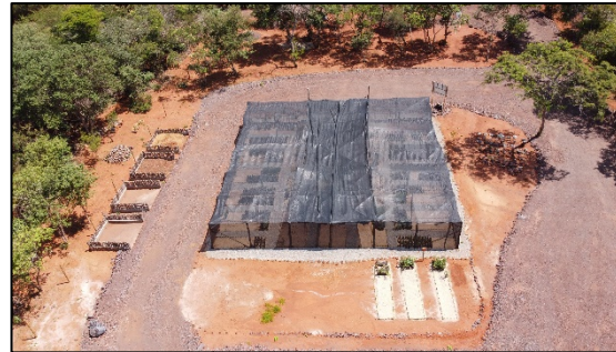
Nursery & Environmental Facility
