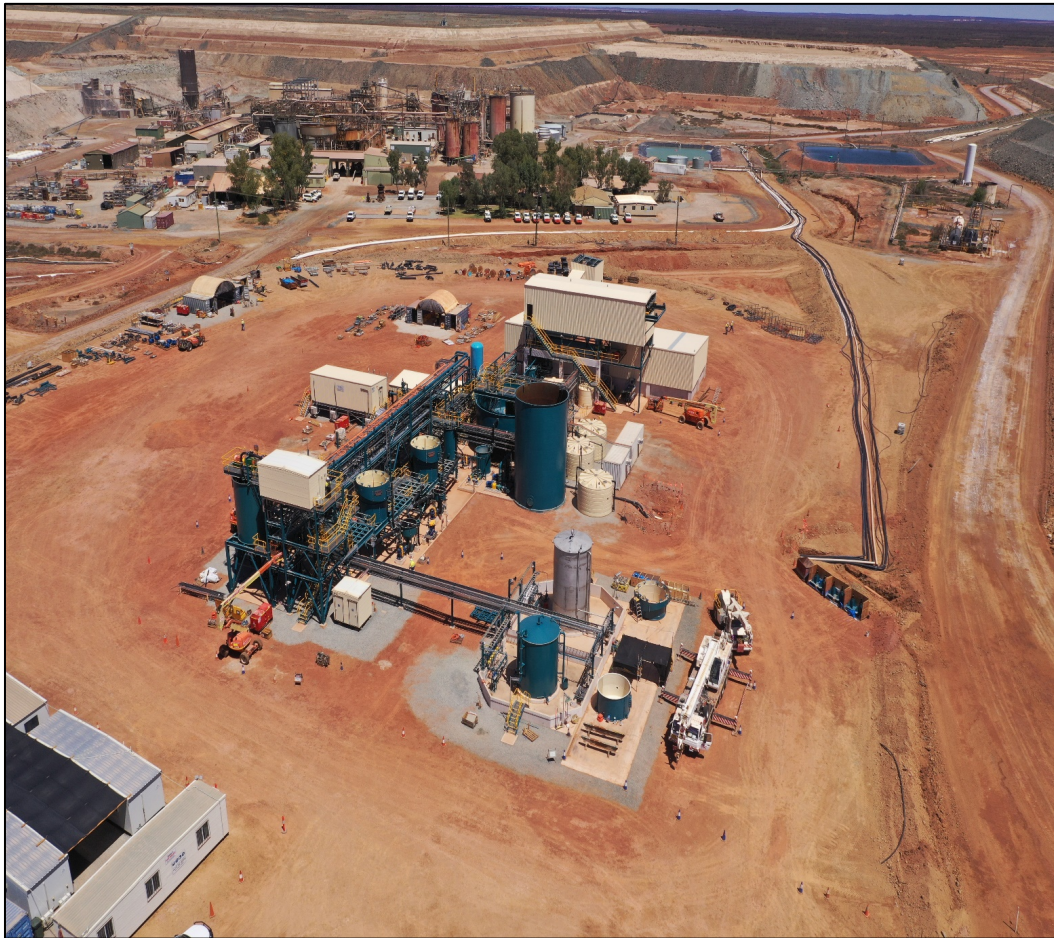
Figure 1: Wiluna Mining concentrator 90% complete and to be commissioned in December 2021 with existing plant in the background.
