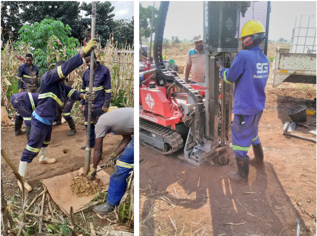
Figure 15 & 16: Field drilling and sampling activities.
