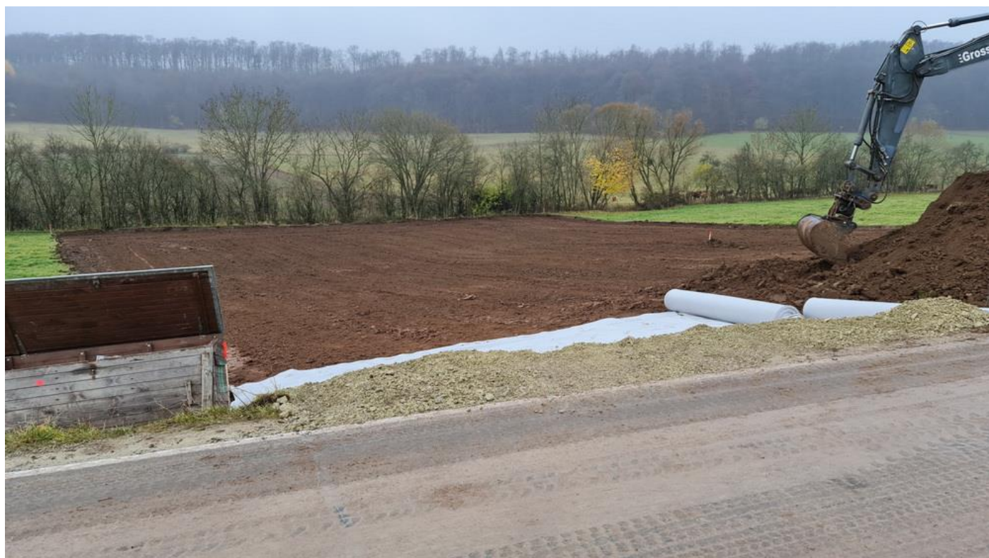
Figure 3: Top soil removed for storage from drill pad at OHM-02.
