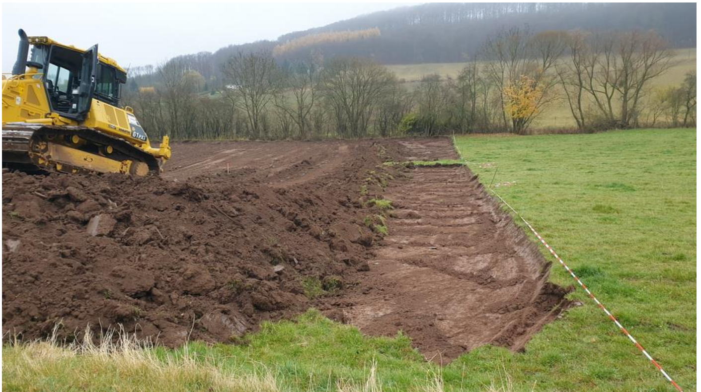
Figure 2: Breaking ground at drill pad OHM-02, week 46 2021
