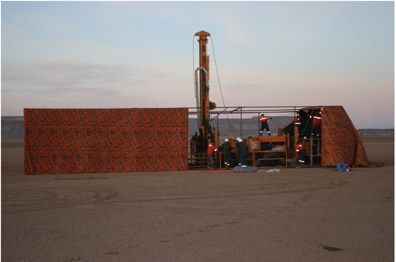
Figure 2: Preparation for Winter Drilling
