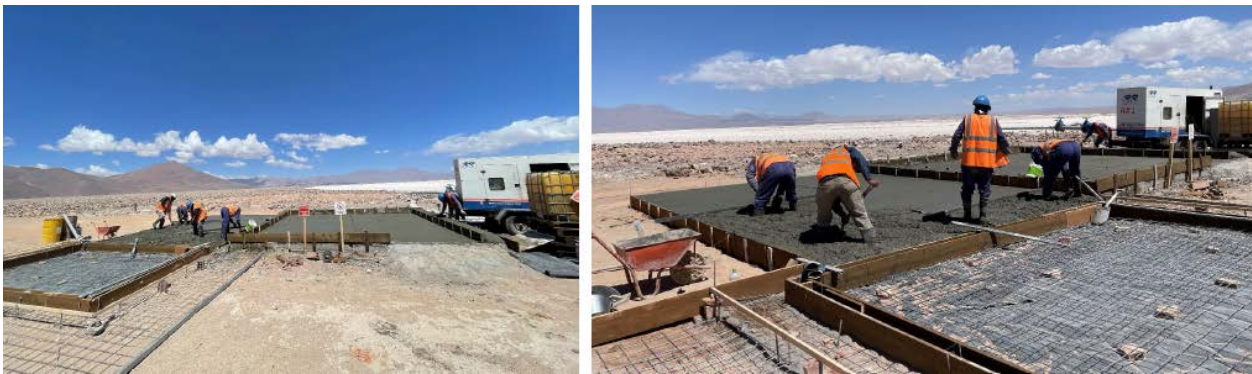
Figure 4. Rincon Lithium Project – 2,000tpa Operation Site Works
