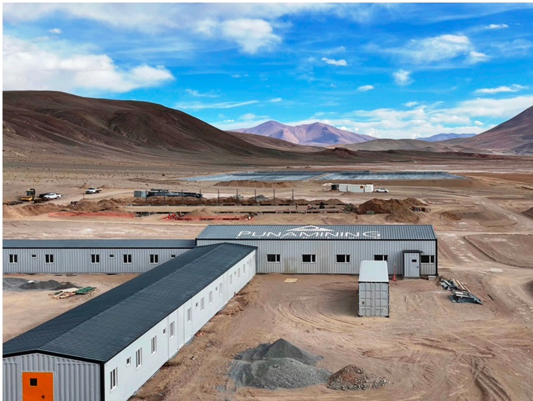
Figure 2. Rincon Lithium Project – 2,000tpa Operation Site Works
