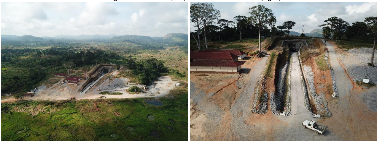
Figure 2. Box Cut (left) and Portal Entrance (right)
