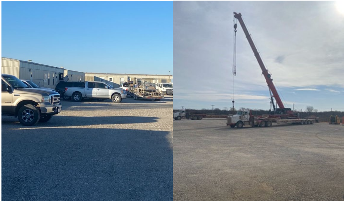
Figure 2: Rangers Well, Stephens County, Oklahoma, Equipment arriving on location
