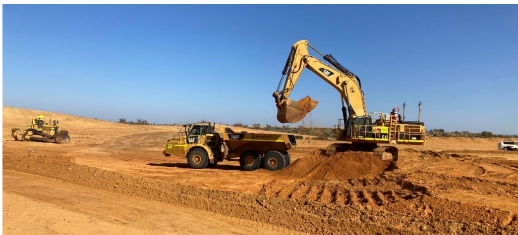
Figure 1 – Breaking ground at Ambassador North pit (11 December 2021)
