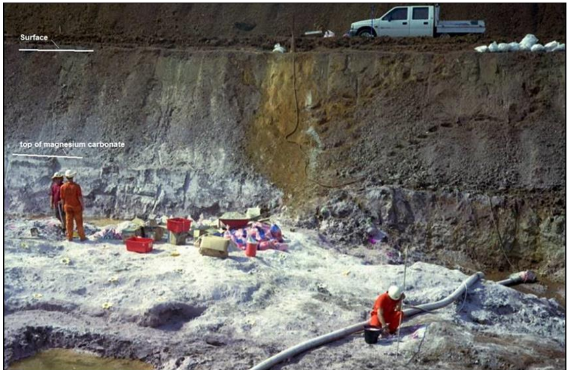
Figure 2 Test mining of magnesium at Winchester during the wet season (preparing to blast Level -1)
