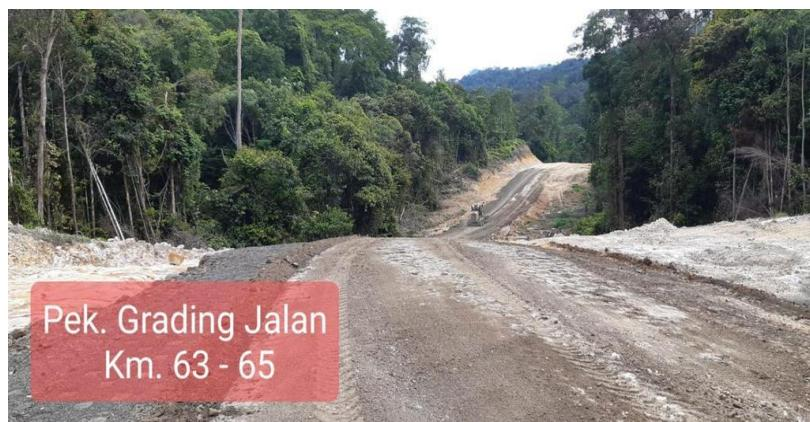
The above photos show that even after heavy rain the road foundation stands up to heavy traffic. After crushed gravel is applied the road will be an all weather road suitable for a mine operating 24 hours a day throughout every month of the year.
