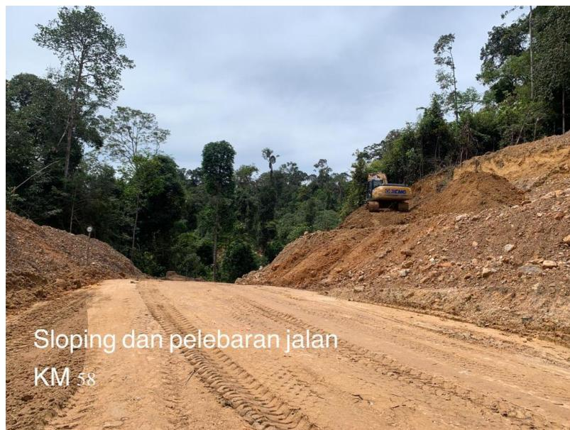
Road upgrading is now in the last 10km before the Mohing River from km 60 to km 70. First task is cutting to grade, then widening and finally grading and compaction to the final profile. This should be completed by the time the Mohing bridge has been completed.
