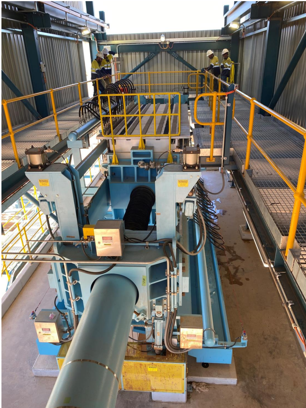
Figure 7: Product Filter Press Commissioning
