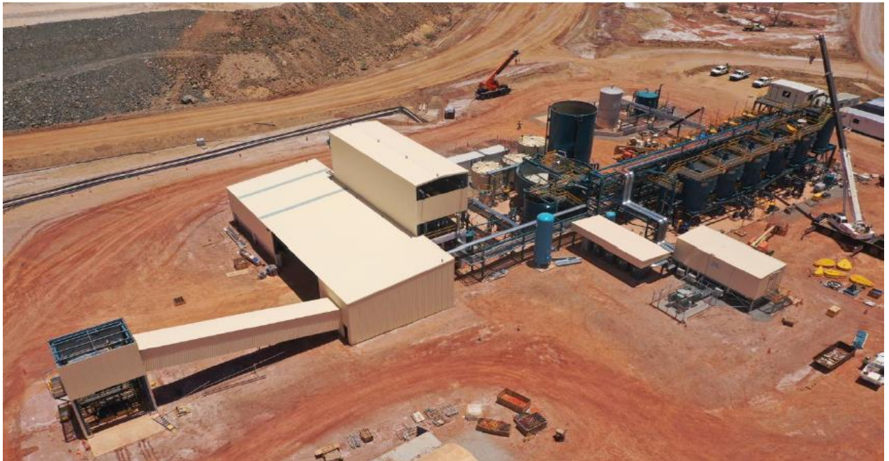
Figure 1: Aerial shot of the Concentrator prior to commissioning
