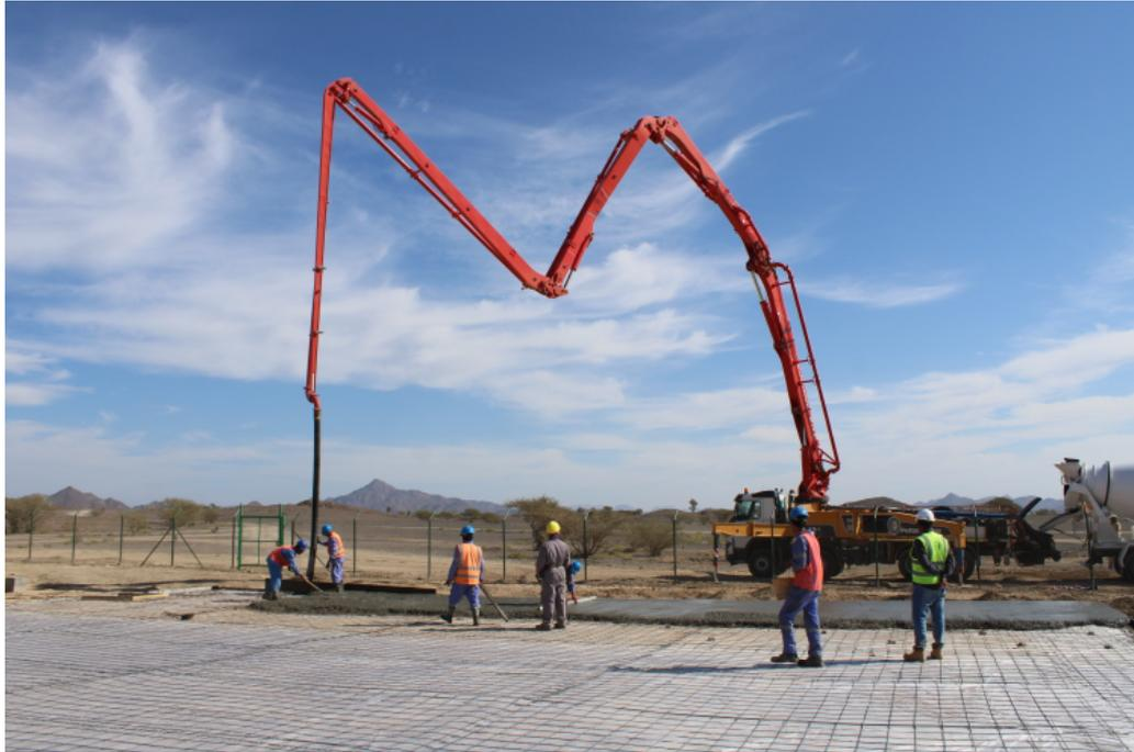
*Picture 3: Dining area ground slab casting*
