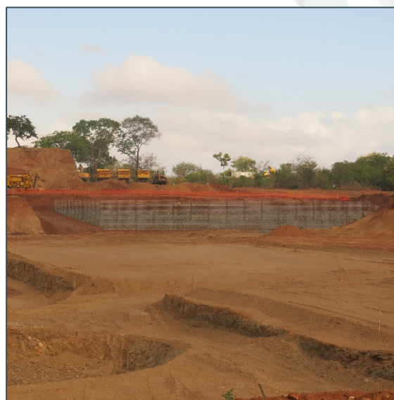
Figure 4: ROM Retaining wall (Terra Trel wall) as of 06 December 2021.
