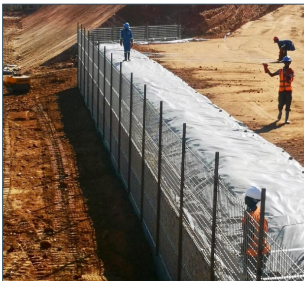
Figure 4: ROM Retaining wall (Terra Trel wall) as of 06 December 2021.
