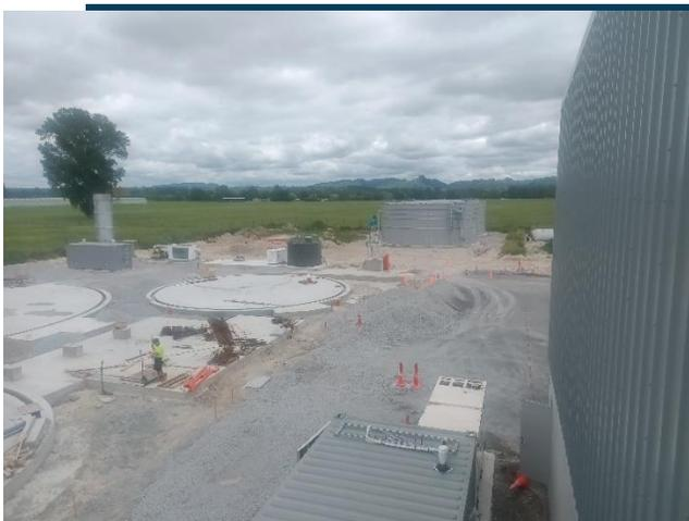
*Image 1: Slab formed by the principal in preparation for AD tank installation*
