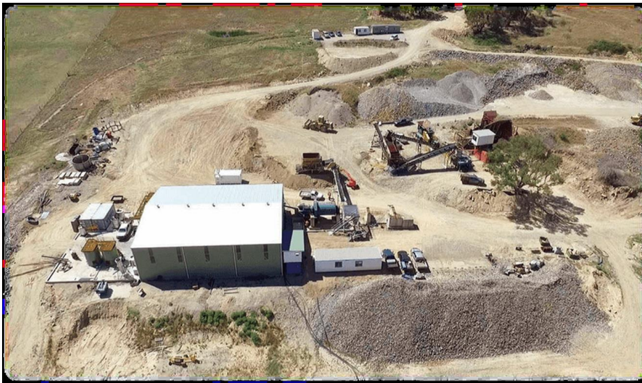
Plant looking south with Adelong Township in the Background
