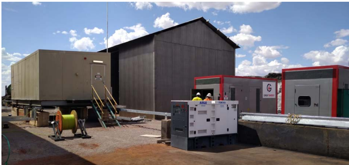
Main motor control room, two of four contract diesel generators and one small ancillary generator.
