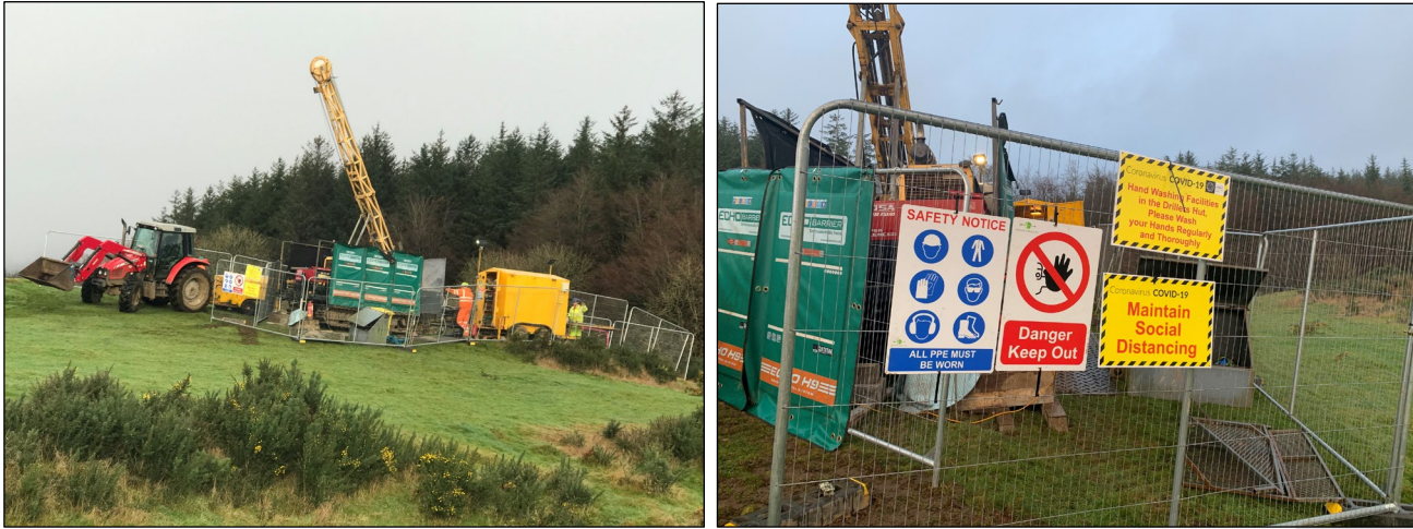
Figure 2: Drill rig in operation on hole 4.
