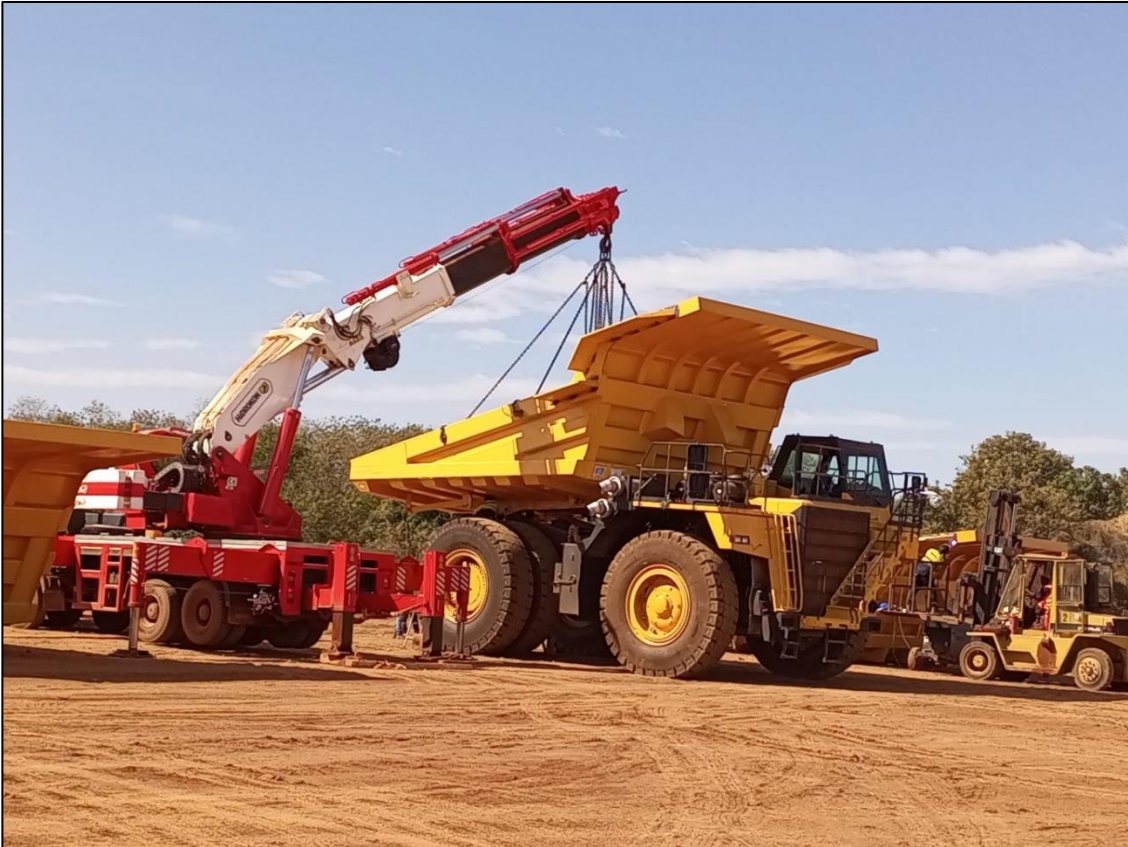
New Komatsu 785 haul truck being assembled onsite at Morila
