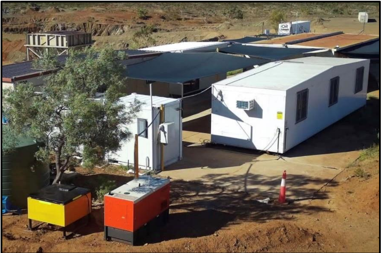
Image 8. Mt Freda office complex.
