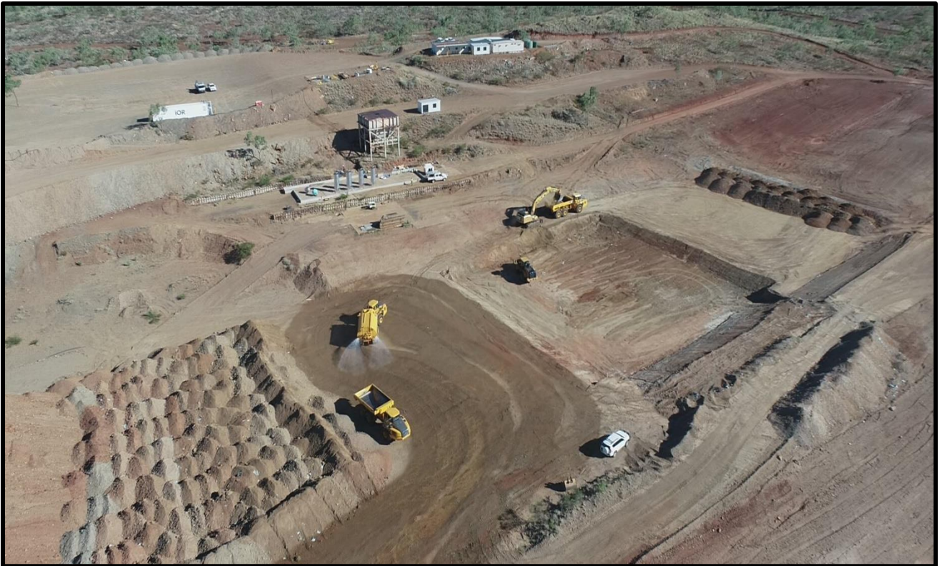
Image 2. Mt Freda Office Complex in the background, Process Plant in the midground and the PLS in the foreground.
