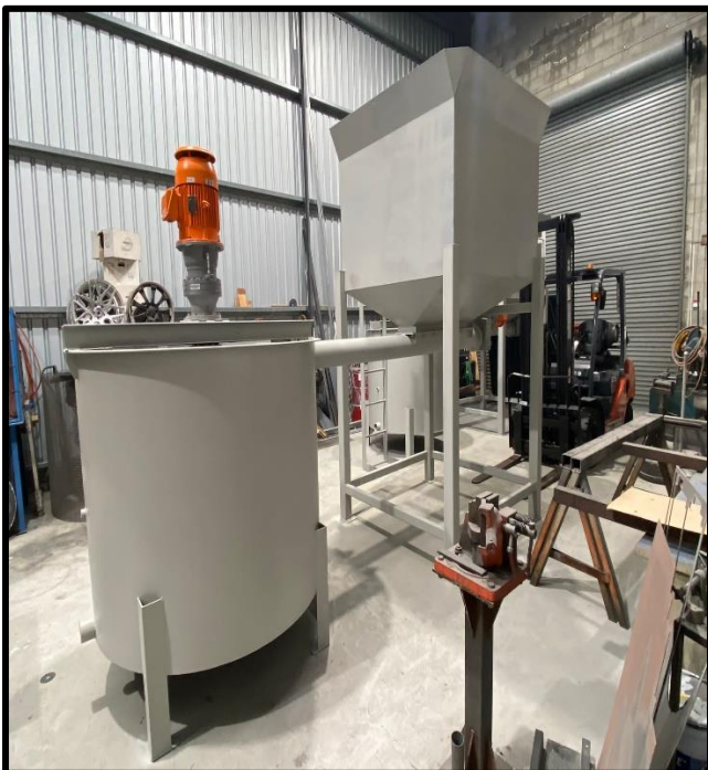
Image 5. Cyanide handling and mixing circuit.
