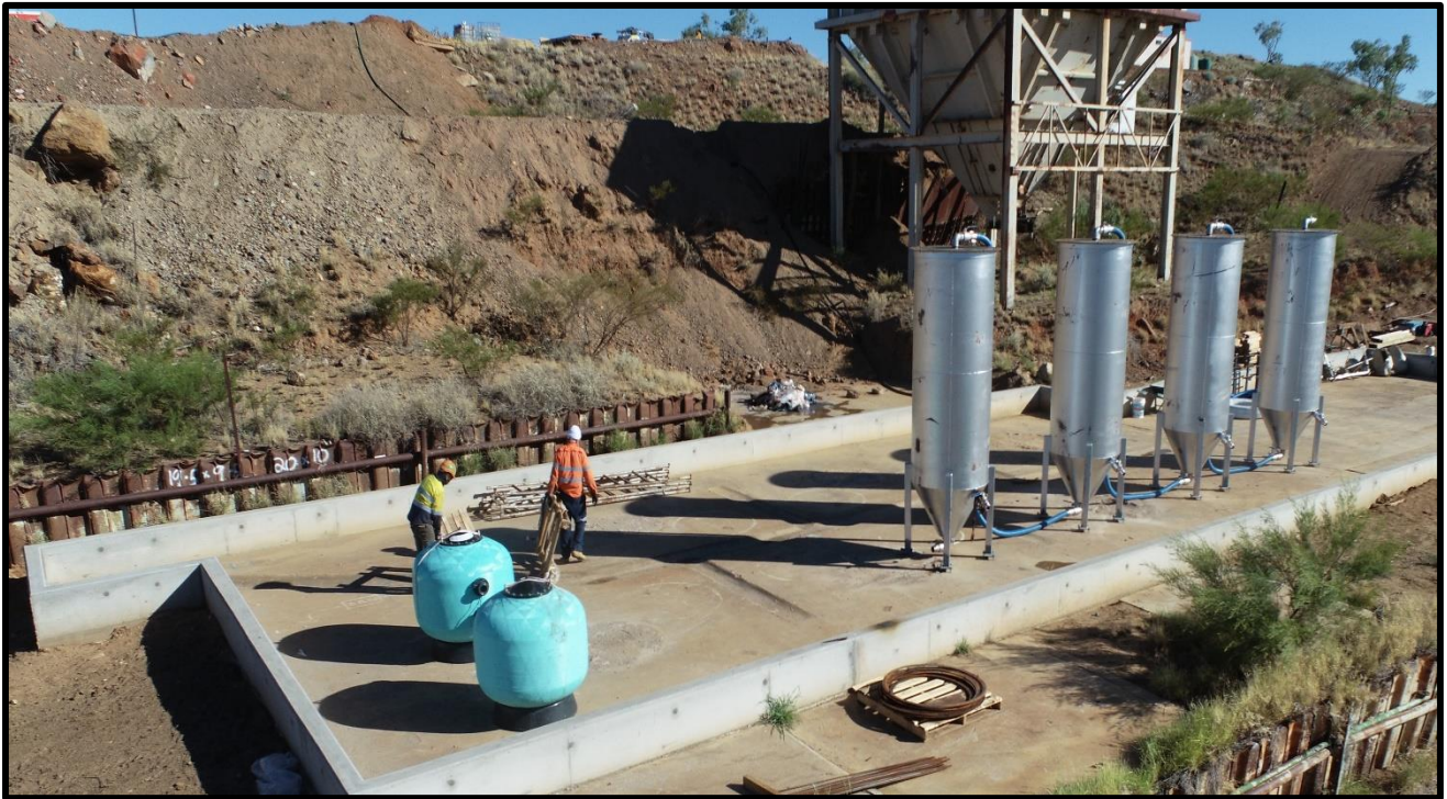
Image 4. Mt Freda Gold Complex Process Plant incorporating the four 2 tonne activated carbon columns.
