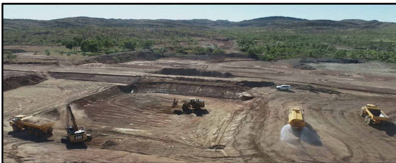
Image 1. Construction of the Pregnant Liquor Solution (PLS) pond has commenced.
