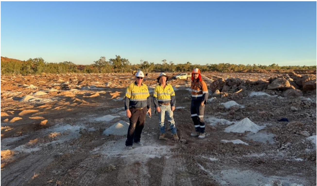
Figure 9. Inspecting blast holes at Anthill east pit prior to loading explosives.
