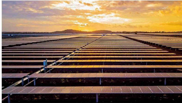
Figure 7 - Merredin Solar Farm (central inverter system, single axis tracked), Western Australia
