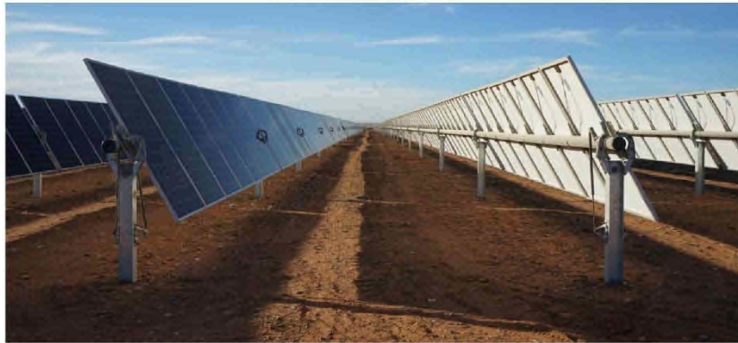
Figure 12 - Single Axis 1P Tracker example
