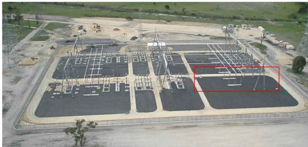
Figure 19 - LWT from south. Bay 924 can be populated to configure LWT as a secure 5-switch mesh
