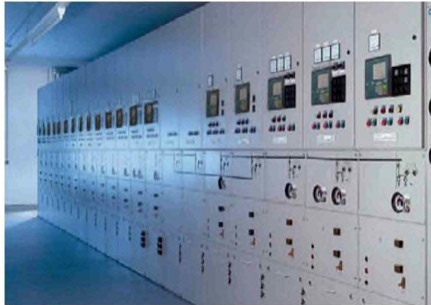
Figure 15 - Typical 33kV GIS collector switchboard (Siemens 8DA10)
