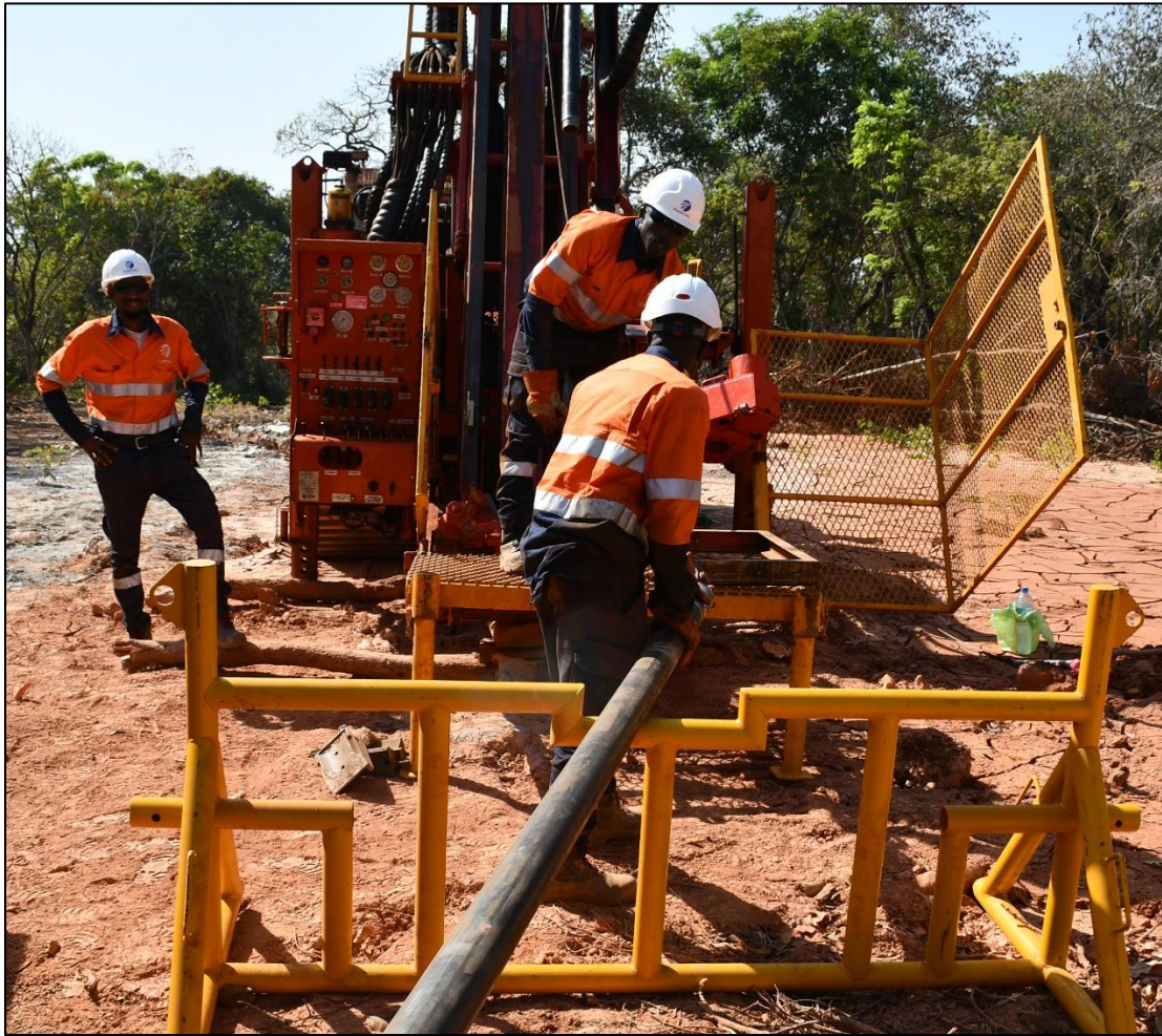
Figure 4 – Diamond Drilling in progress at the NE Bankan Deposit, Guinea
