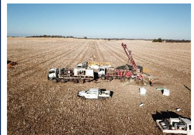
Drill rig at Moora
