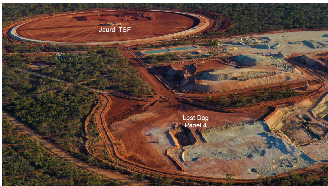
Jaurdi TSF – Earthworks 75% complete
