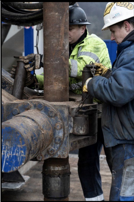
Photos 1 – 4 clockwise: Drill rig at Ohmgebirge (1) with installation of the 13 3/8” conductor casing (2). Coring will begin at a depth of 525m from surface. Drill rod handling (3) and public information boards (4) are also depicted.
