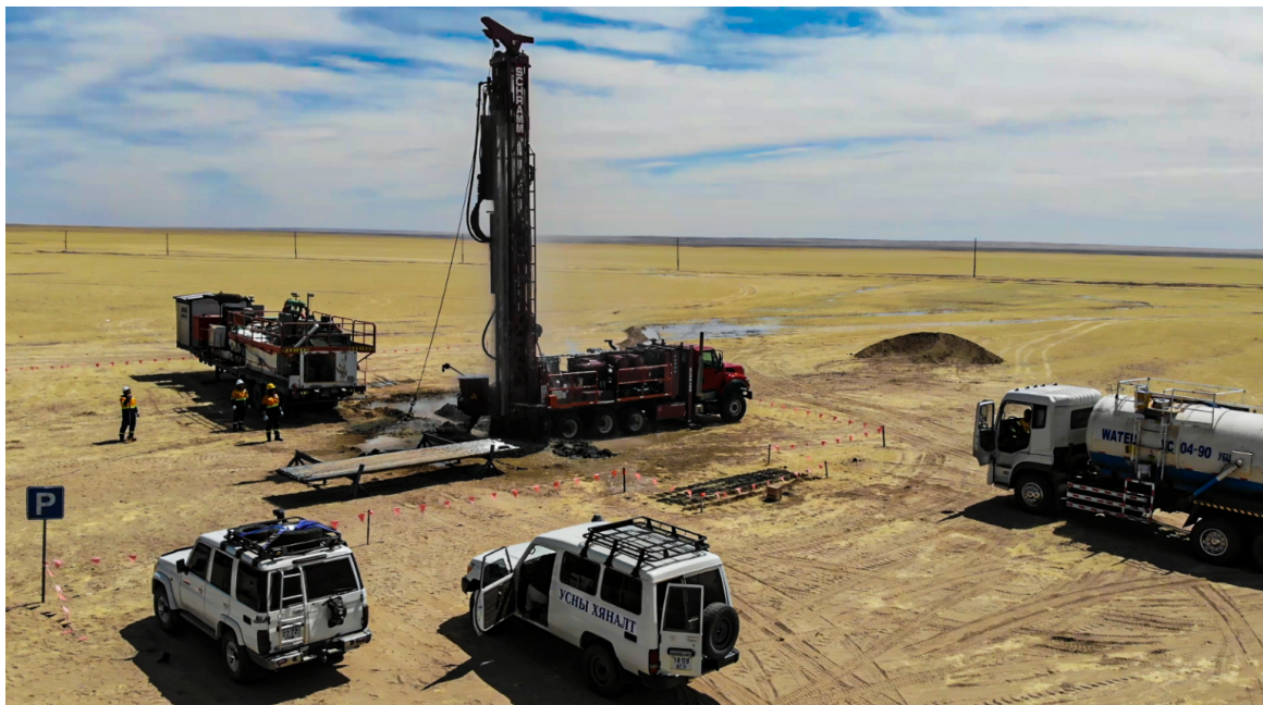
ErdeneDrilling's water drilling operations in the Gobi region
