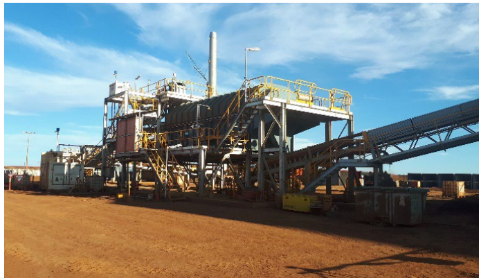
Concentrate Dryer construction completed with pre-commissioning
