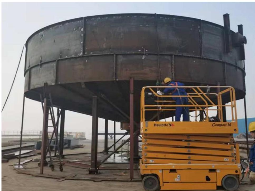
**Figure 6** – Concentrate thickener fabrication.
