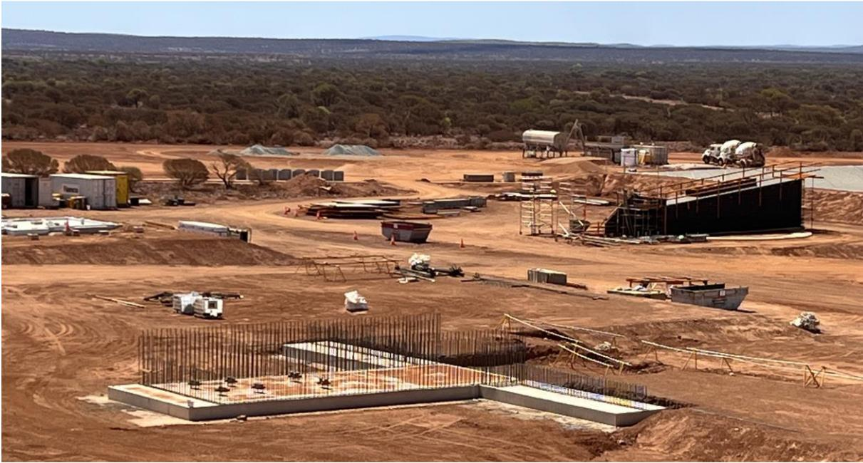
**Figure 7** – Processing plant site works showing crusher, screening, and ore storage foundations.
