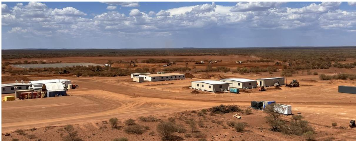
**Figure 4** – Construction offices, mine administration, and mining contractor buildings in place. Completed plant site earthworks in the foreground and civil construction occurring in the background on site power station earthworks.
