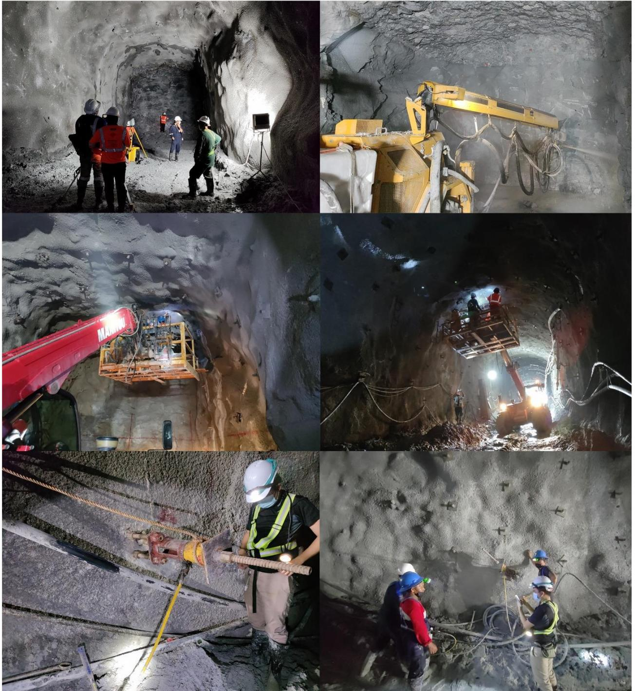
**Figure 1. Decline Development Cycle** – Face Drilling & Blasting, Mucking, Scaling, Initial Shotcrete Spraying (Batching), Survey & Mapping, Rockbolt Installation, Final Shotcrete Spraying, and QAQC Activities (Pull-out and Thickness Testing)
