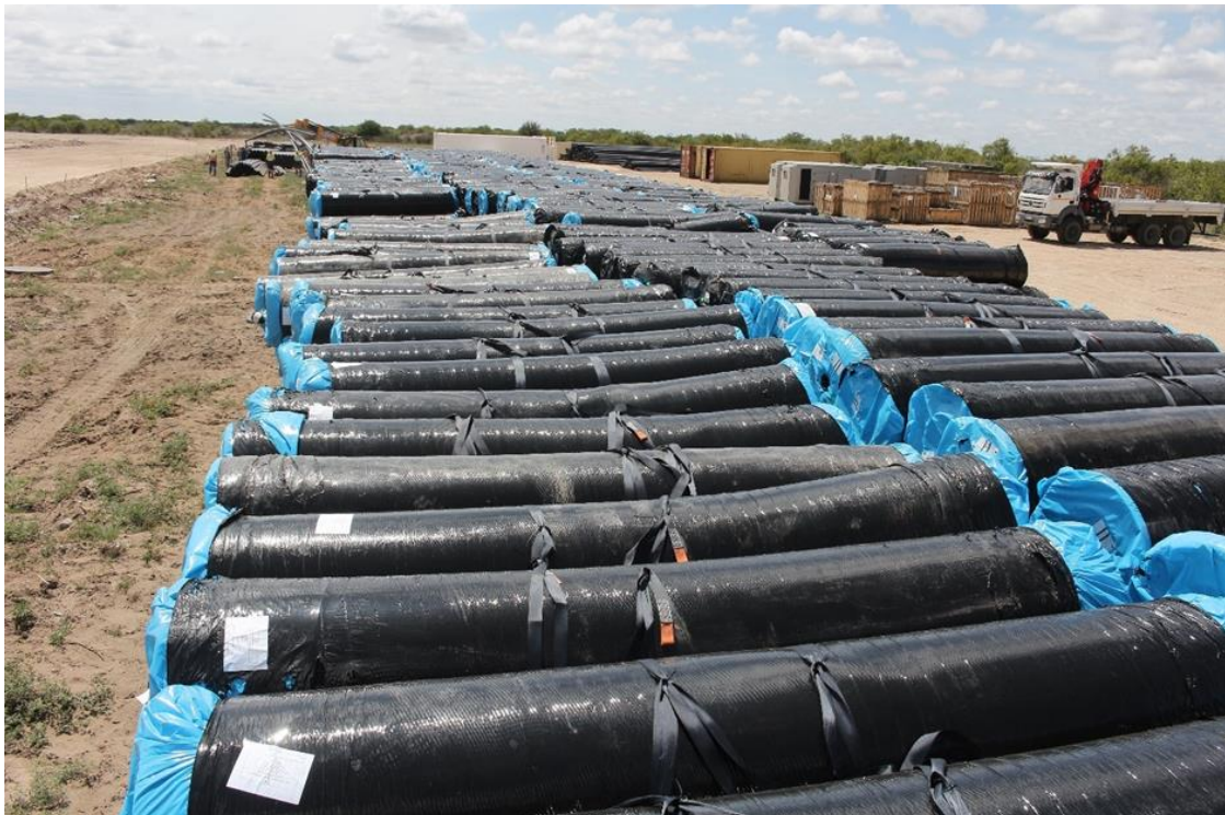
Figure 6. TSF liner deliveries commenced
