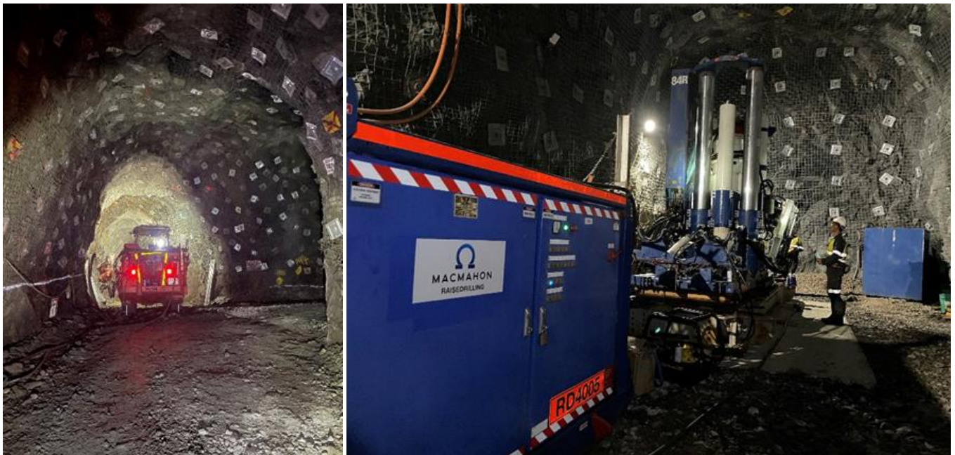
Northern Operations – L to R - Durkin Decline and Raisebore Chamber setup.
