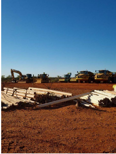
Access road fleet at Yangibana
