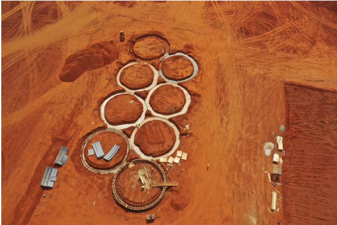
Figure 9: CIL Ring Beams and Rebars and Formwork in progress
