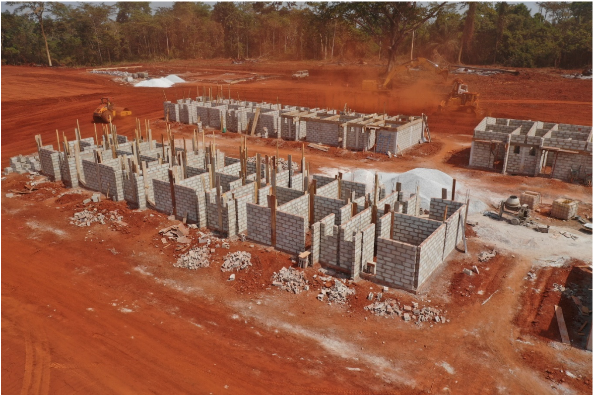
Figure 8: Camp accommodation units under construction
