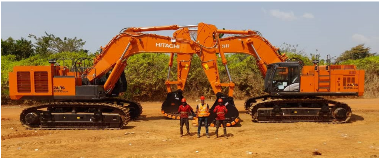
Figure 11: Tietto's 2 newly acquired excavators on site
