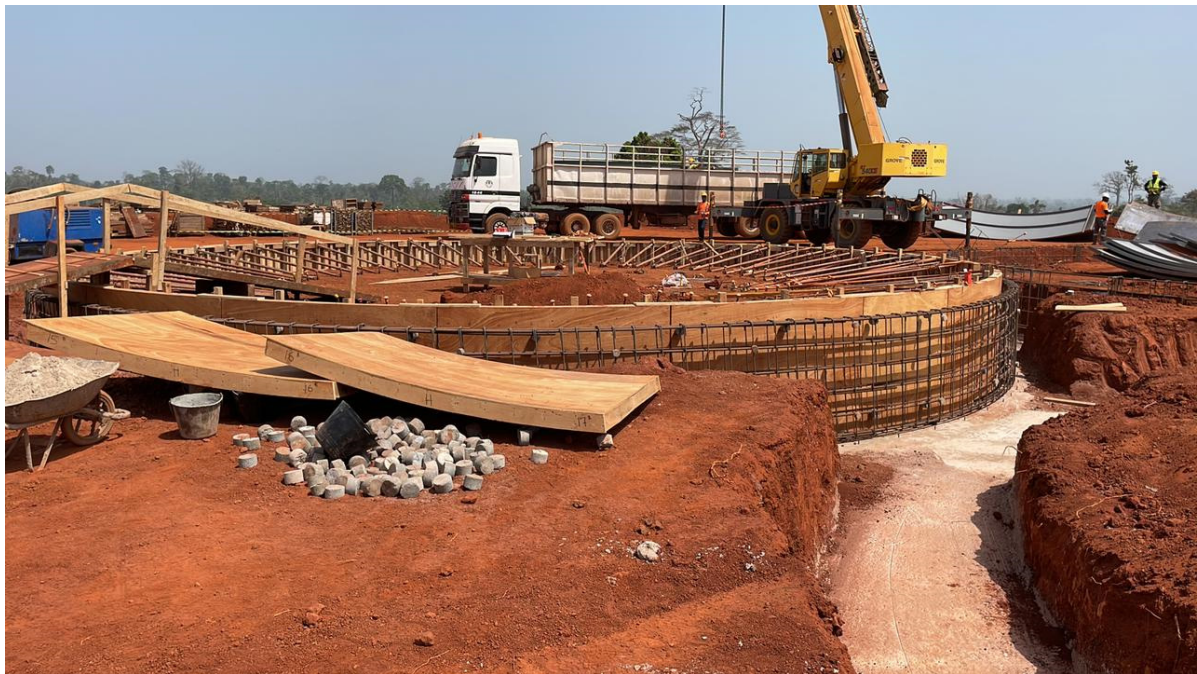
Figure 1: CIL Rebar and formwork in progress
