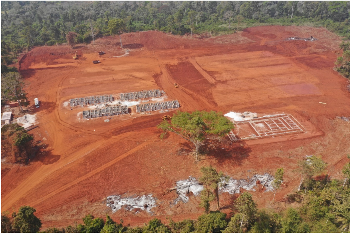
Figure 7: Mine camp in construction
