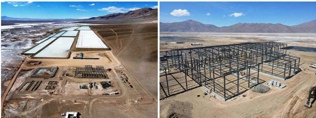
Figures 4-5. Rincon Lithium Project – 2,000tpa Operation Site Works in Progress
