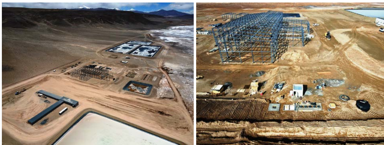
Figures 2-3. Rincon Lithium Project – 2,000tpa Operation Site Works in Progress
