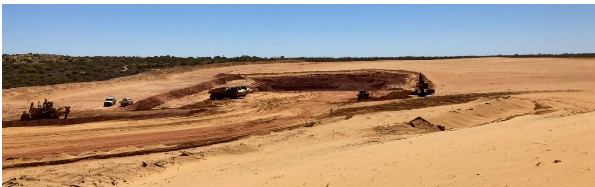
Figure 1 – Ambassador North pit ramp excavation
