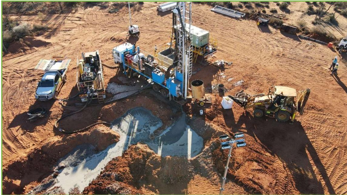
Figure 2: Borefield drilling
