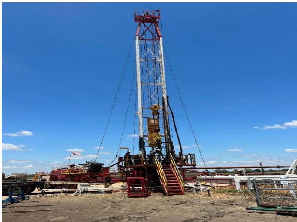
Image of Myall Creek-2 location during workover operations in January 2022.
