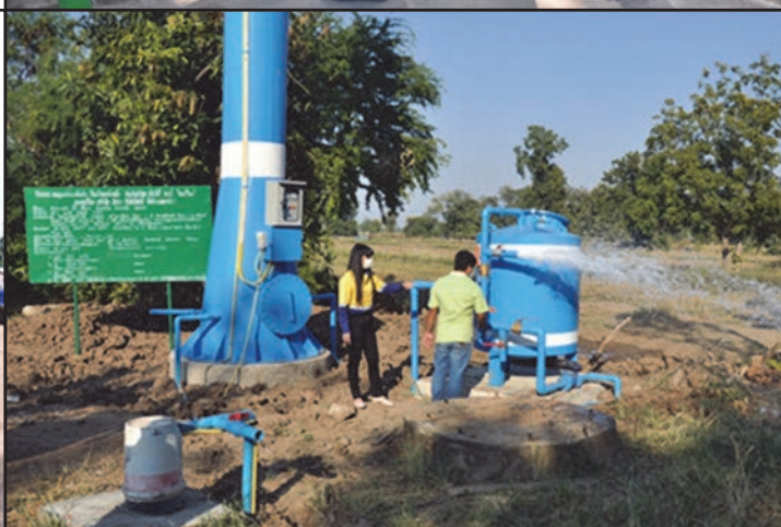
(Above). Water supply systems were upgraded to meet the increasing water-use needs of the Chatree Community. Works included (at left) installing solar power to reduce power costs and support Thailand's Green Economy plan along with (at right) the installation of new water pumps, rust filters and piping.
