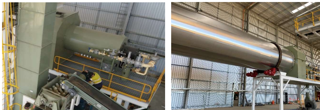
Figures 1 and 2. Stantil Engineering Kiln installed onsite.
