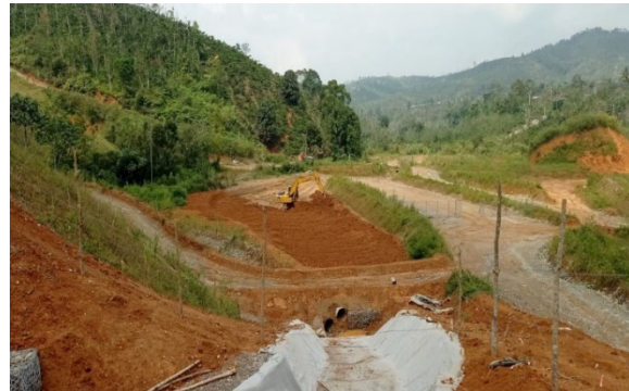
Spreading soil at ex ore stockpile Talang Santo
