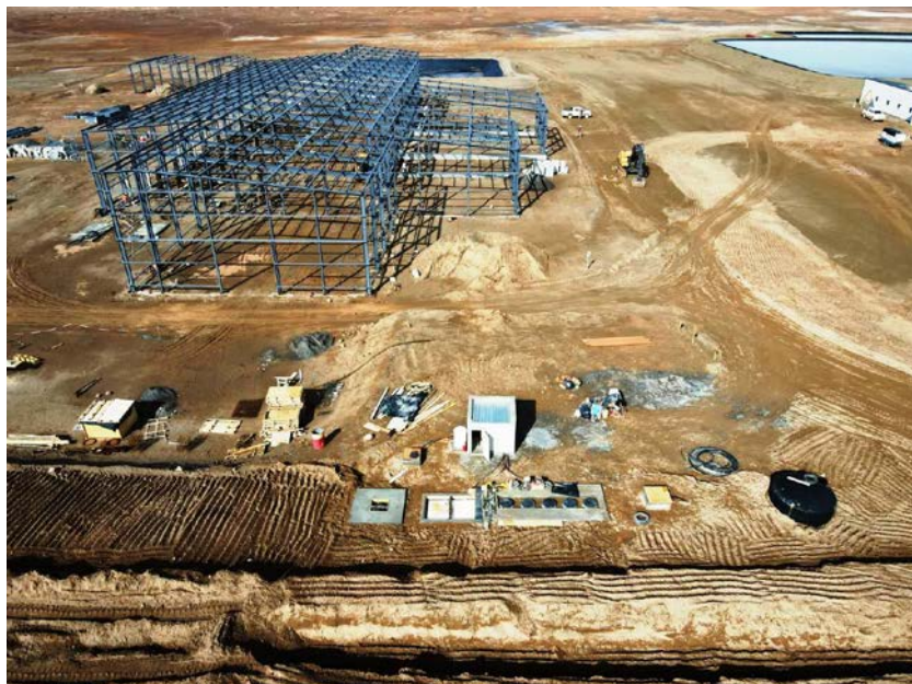
Figure 6. Rincon Lithium Project – 2,000tpa Operation Site Works
