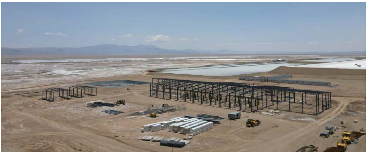
Figure 2. Rincon Lithium Project – 2,000tpa Operation Site Works
